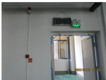
Exit sign, emergency light and fire alarm.JPG
